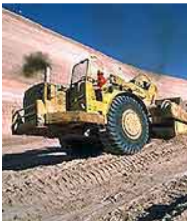
Figure 2-3: Heavy Equipments for clearing and grading
