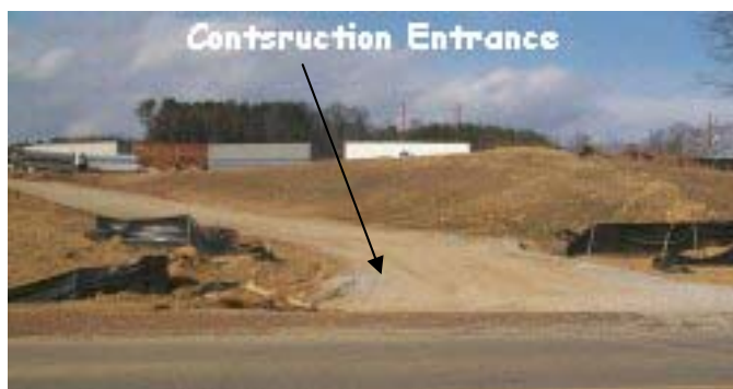
Figure 2-2: Construction site entrance
